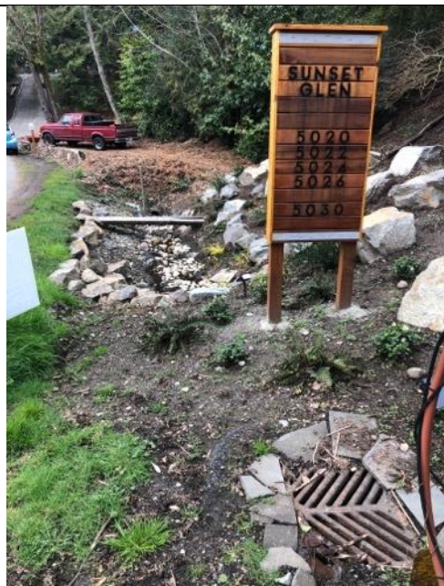
Photo 8. View of the drain grate and area where the piped watercourse connects with the open and possibly daylighted section of the Type Ns stream, looking north. Photo taken 3-17-22.
