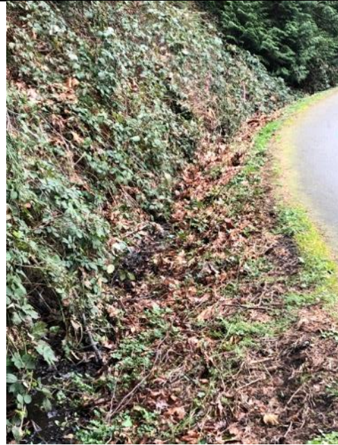
Photo 4. View of Wetland A within Ditch 1, looking south. Photo taken 3-17-22.
