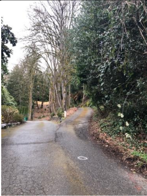
Photo 3. View of driveway access road at north end of Project Site which directs stormwater to Ditch 1/Wetland A.
